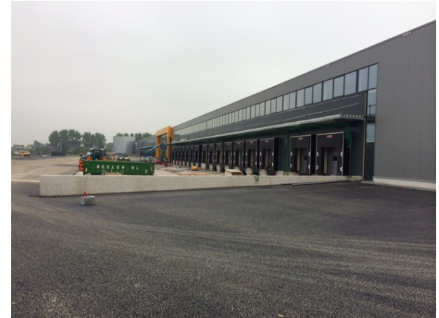
Distribution centre Landsingerland under construction
